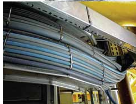
Ball-Lok Ties are used to secure cables in cable trays.
